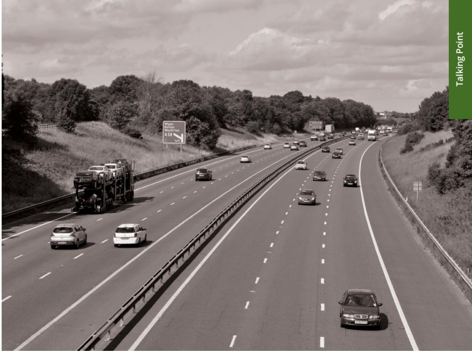
▲ Carillion and Kier were working as a joint venture to deliver the M6 Smart Motorways scheme on behalf of Highways England
