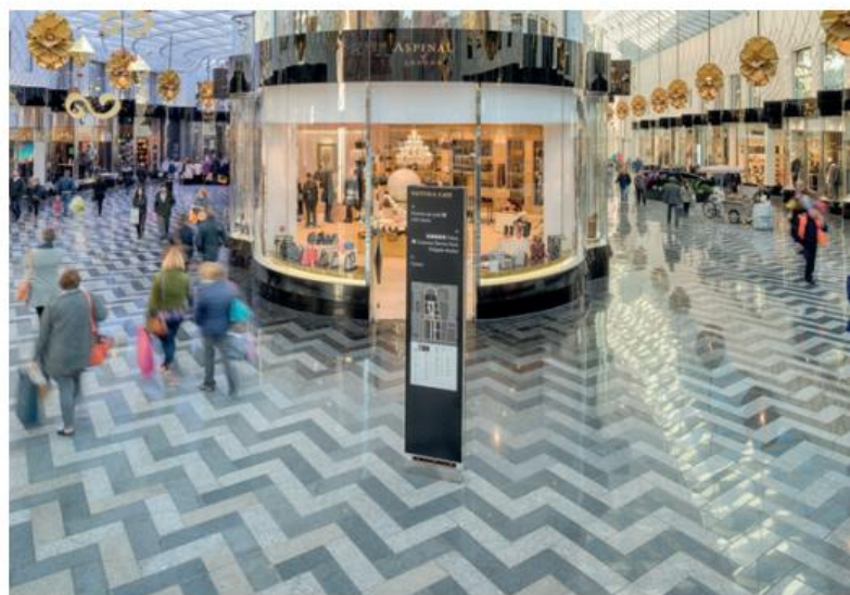
▲ All 3000m 2 of polished granites and specialist bespoke granite staircase features were checked for quality of cut, colour blend and durability before being shipped to Yorkshire for the new Victoria Gate retail development in Leeds
