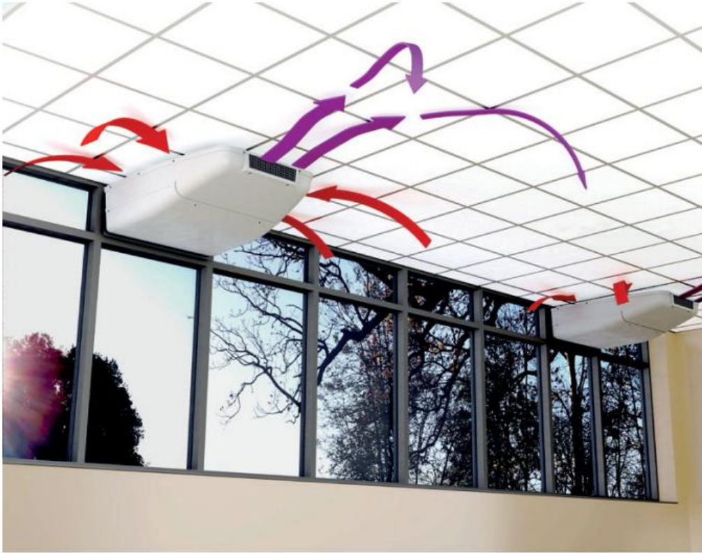
▲ Passivent's Hybrid Plus2 Aircool ventilators in situ
