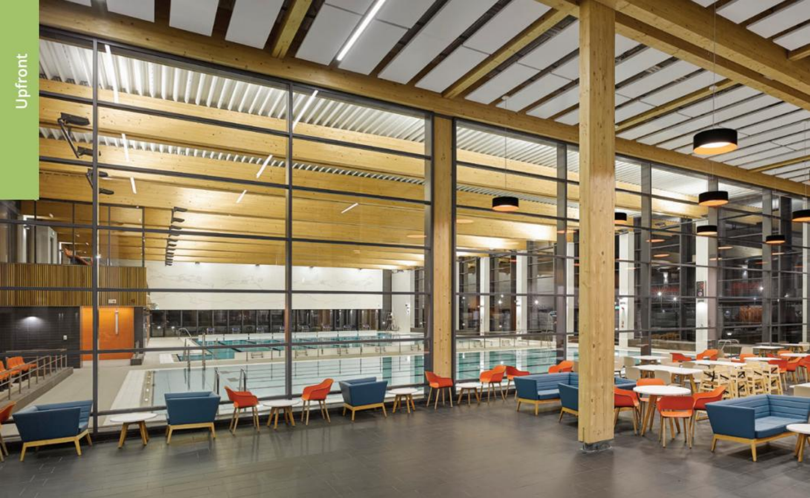
▲ The building demonstrates that high-quality design, with exceptional daylight and openness, can be achieved in tight timescales
